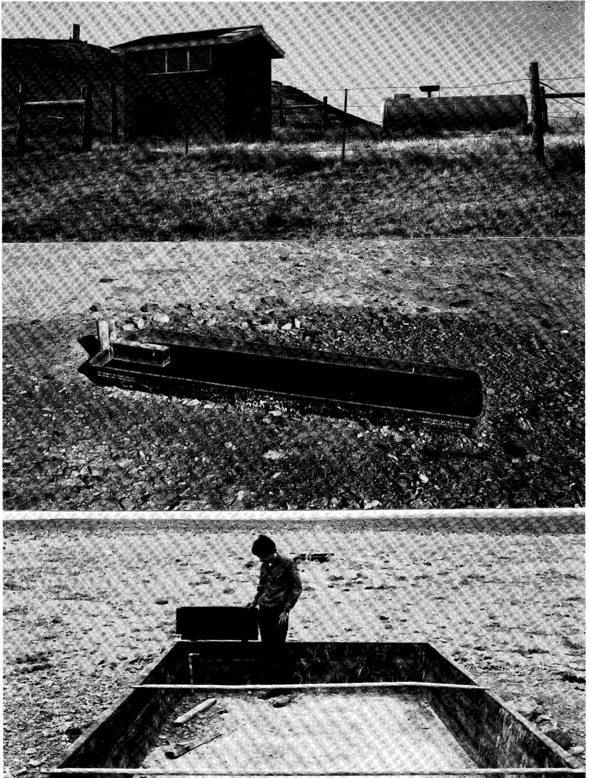
Figure 26.--A second type of water system uses a well and butane-operated pump, a metal storage tank on the hill (top), and pipeline to troughs (middle). The large shallow trough (bottom) stores water and permits cattle to escape if they fall into the trough.
